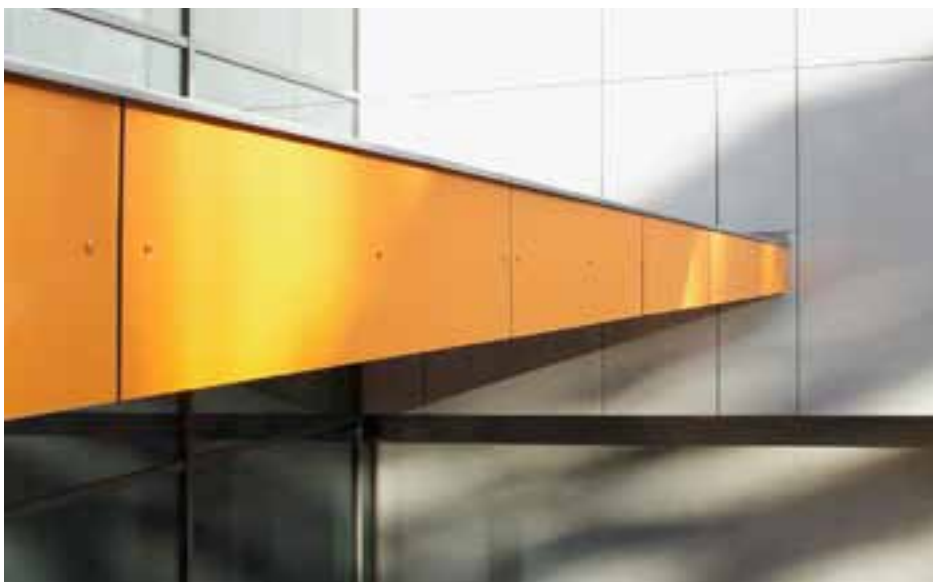
The reinforced concrete was thermally insulated and clad with façade panels. The glazed connection between the old and the new buildings are implemented as thermally separated aluminium profiles, as all the windows.
