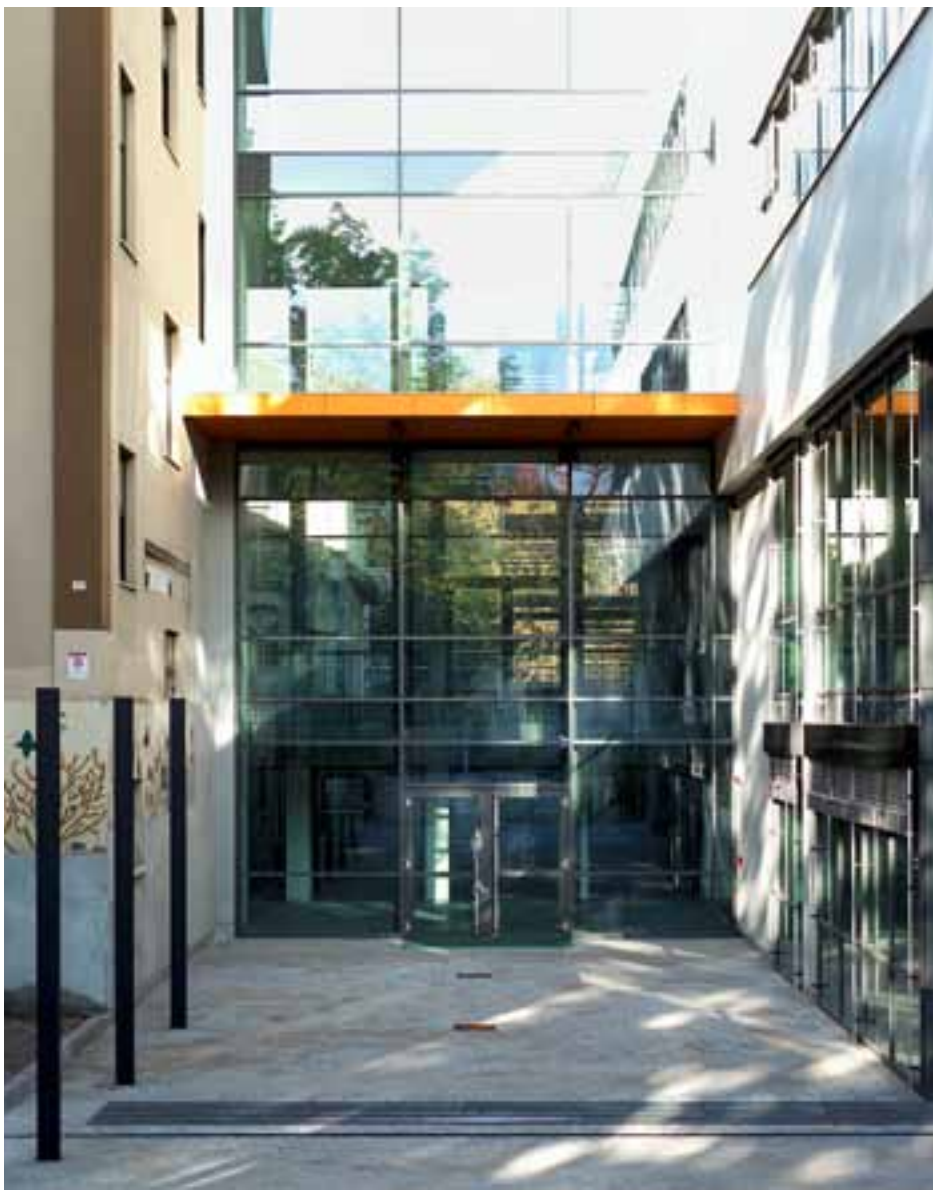
The reinforced concrete was thermally insulated and clad with façade panels. The glazed connection between the old and the new buildings are implemented as thermally separated aluminium profiles, as all the windows.
